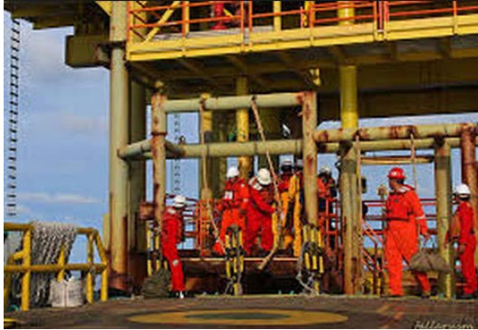
Figure 9. Transferring workers via swing ropes, in the Gulf of Guinea area
