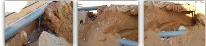
Image: crumbled foggara and water leaks
