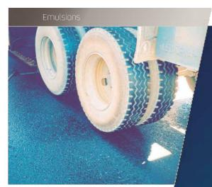
**Thermo-Adhesive Emulsions** are rapid breaking emulsions with special characteristics with regards to adhesiveness between layers, adhesion to the support and little to no sticking to the tyres of the work vehicles.
