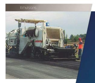
The emulsion C60B5 REC REJUV, specially developed by Repsol for the cold-mix recycling of aged surfaces, is a super-stabilised emulsion, formulated with rejuvenating binders, that meets the General Technical Specifications for Roads and Bridge Works [PG-3] for type C60B7 REC emulsions. This product is specially designed for each project and provides the components lost by the original bitumen on the road as a result of its ageing, restoring its initial characteristics.
