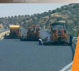
The special bitumens for recycling developed by Repsol are custom-made binders that provide the components that have been lost in the bitumen as a consequence of its ageing, returning it its original characteristics and properties (physical and chemical).
