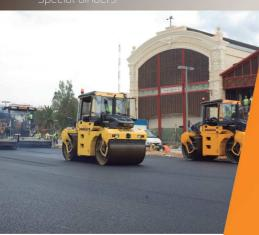
The PMB 45/80-75 F bitumen is a technologically innovative binder obtained through a process of chemical reticulation with a high polymer content, which has a microscopically homogeneous structure and is completely stable in storage.
