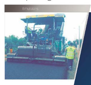
Repsol has developed the medium breaking bituminous mix **C67B3 MBA EFIMUL**, formulated ad hoc for the manufacture of open-graded mixes; storable, able to be handled at room temperature and specifically designed to take advantage of the versatility and mobility offered by the machinery for manufacturing and spreading bitumen slurry.
